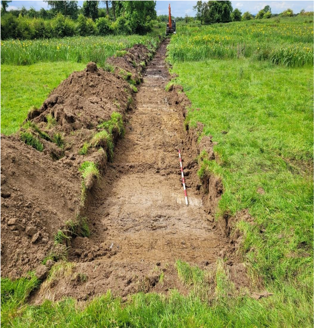
Plate 14: Trench 23, facing southwest.
